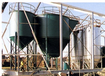
INSTALLATION OF A TREATMENT PLANT CONSISTING OF A SPECIAL PLATE SEPARATOR AND DYNASAND FILTER.
