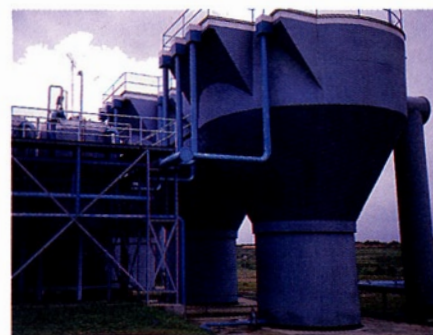
THE JOHNSON LAMELLA SEPARATOR.
