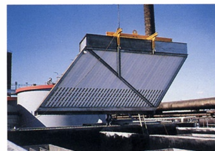
PLATE PACK ASSEMBLIES ARE SUPPLIED READY FOR INSTALLATION.
